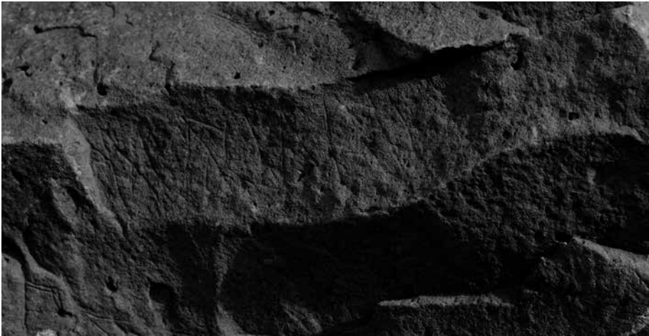
Figura 10. Sector 1, Panel 6. Detalle.
